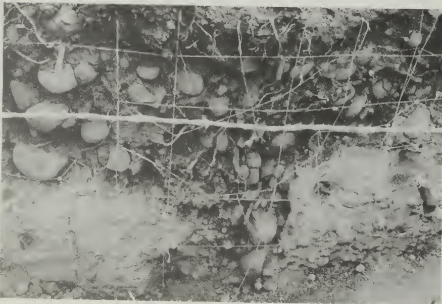
Figure 18. The main fault feature in trench BHT-53 consisting of colluvium overlying weathered conglomerate and a "pseudopaleosol" that is developing contemporaneously in an old shear zone.
